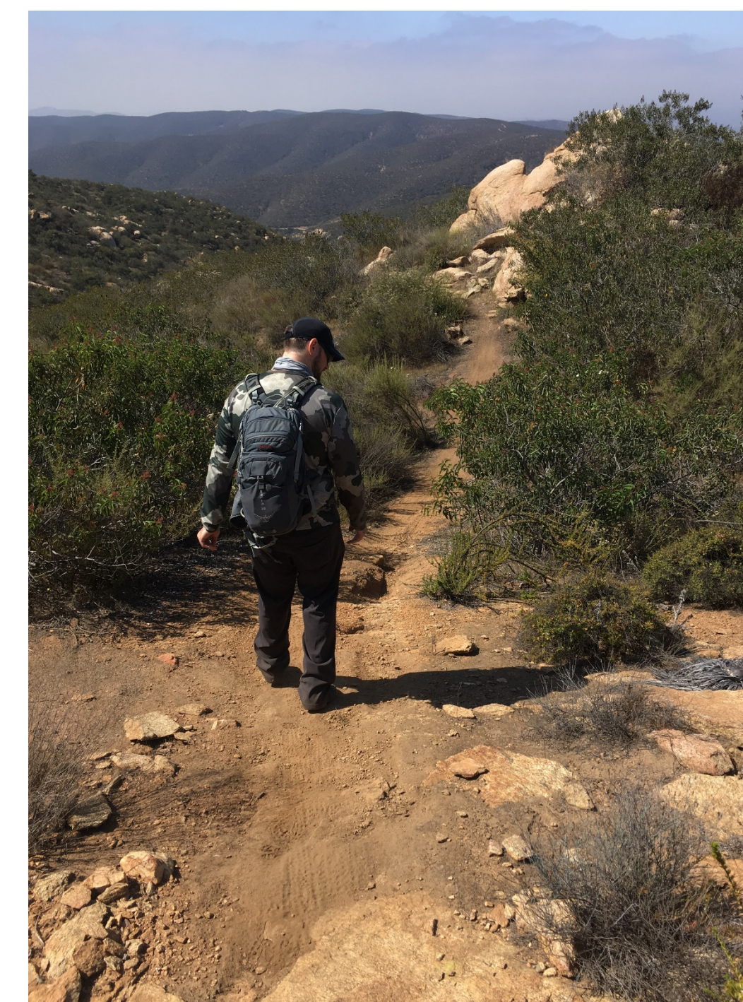
Existing Condition: Eastern Sycamore Canyon 2-4 foot tread width would be maintained Grade ranges from 5-20% along trail
