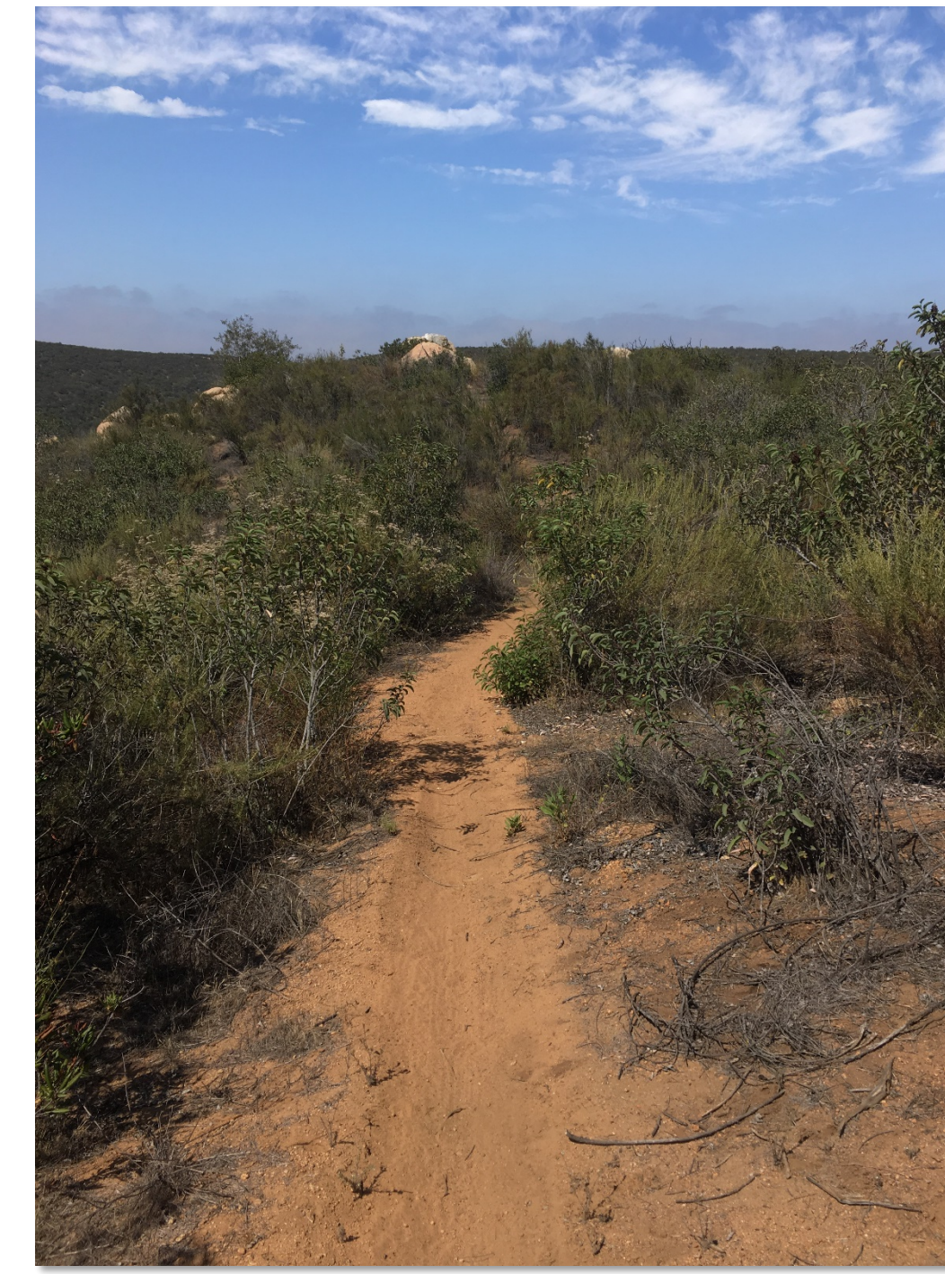
Existing Condition: Eastern Sycamore Canyon 2-4 foot tread width would be maintained Grade ranges from 5-20% along trail
