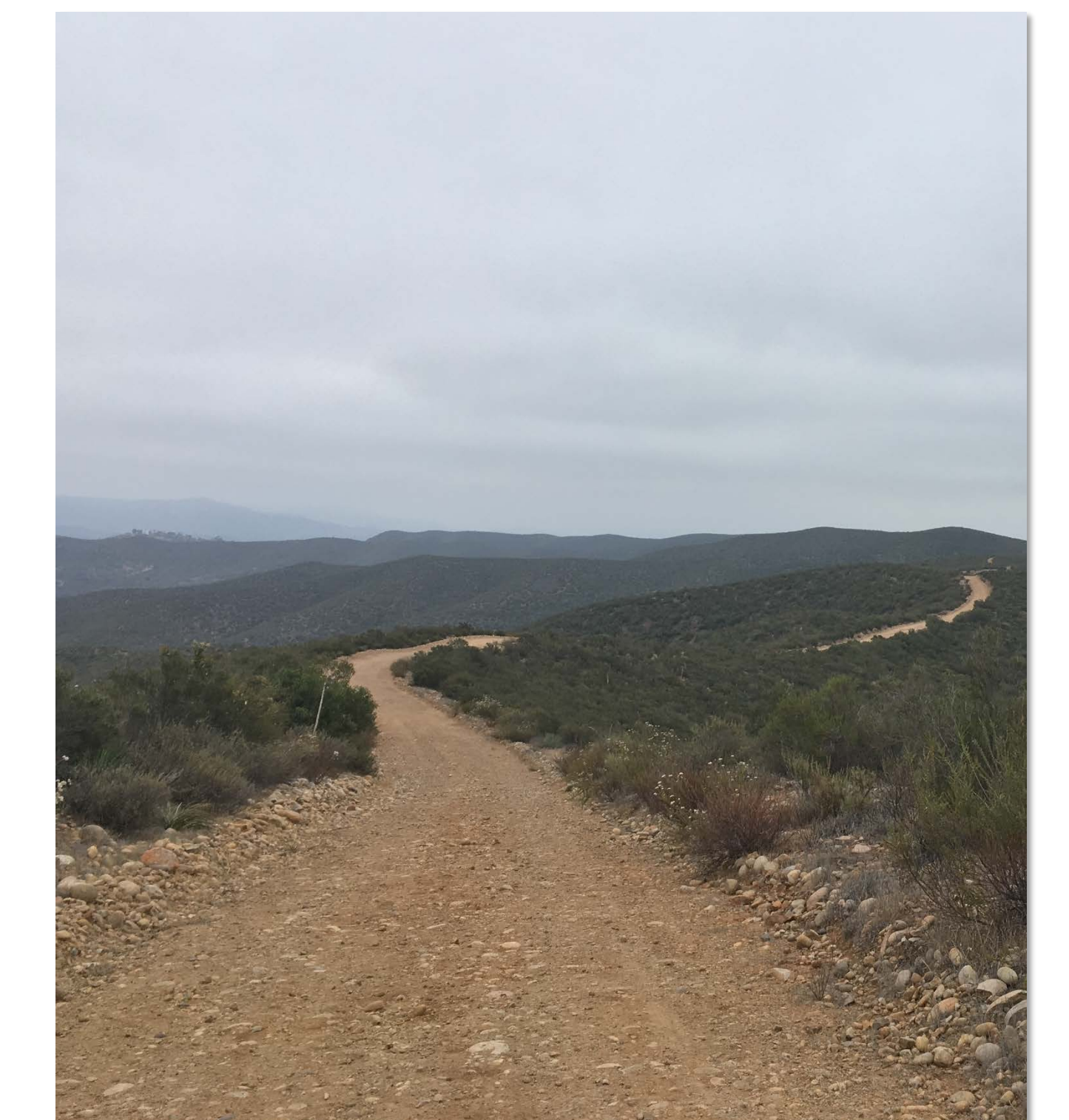
Existing Condition: Slaughterhouse Canyon Trail (CWA Access Road segment) 10-12 foot tread would be maintained, serves as a shared multi-use trail and maintenance access road
