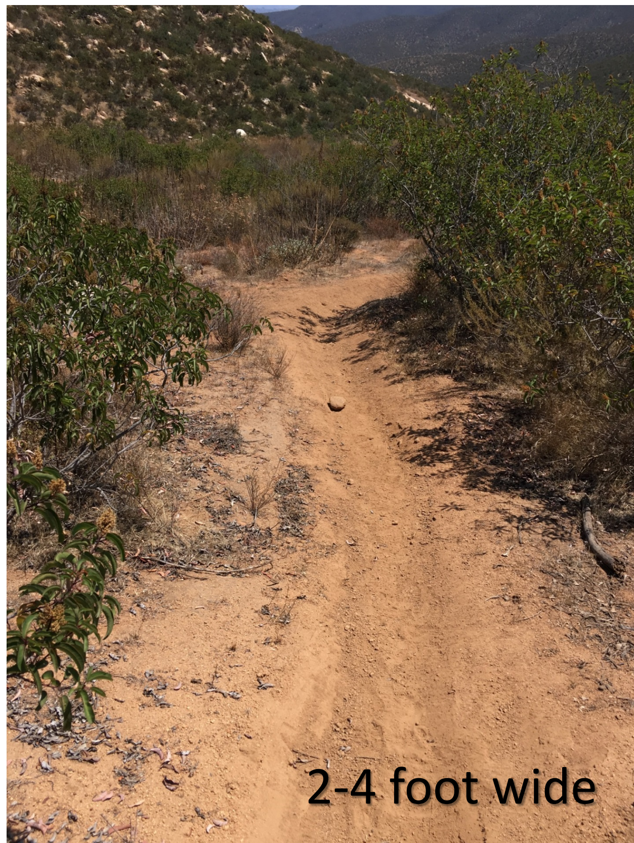
Existing Condition: Eastern Sycamore Canyon 2-4 foot tread width would be maintained Grade ranges from 5-30% along trail
