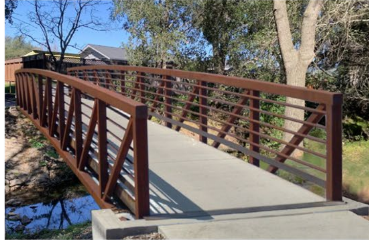
Prefabricated steel pedestrian bridge with non-slip concrete walkway at creek crossings.
