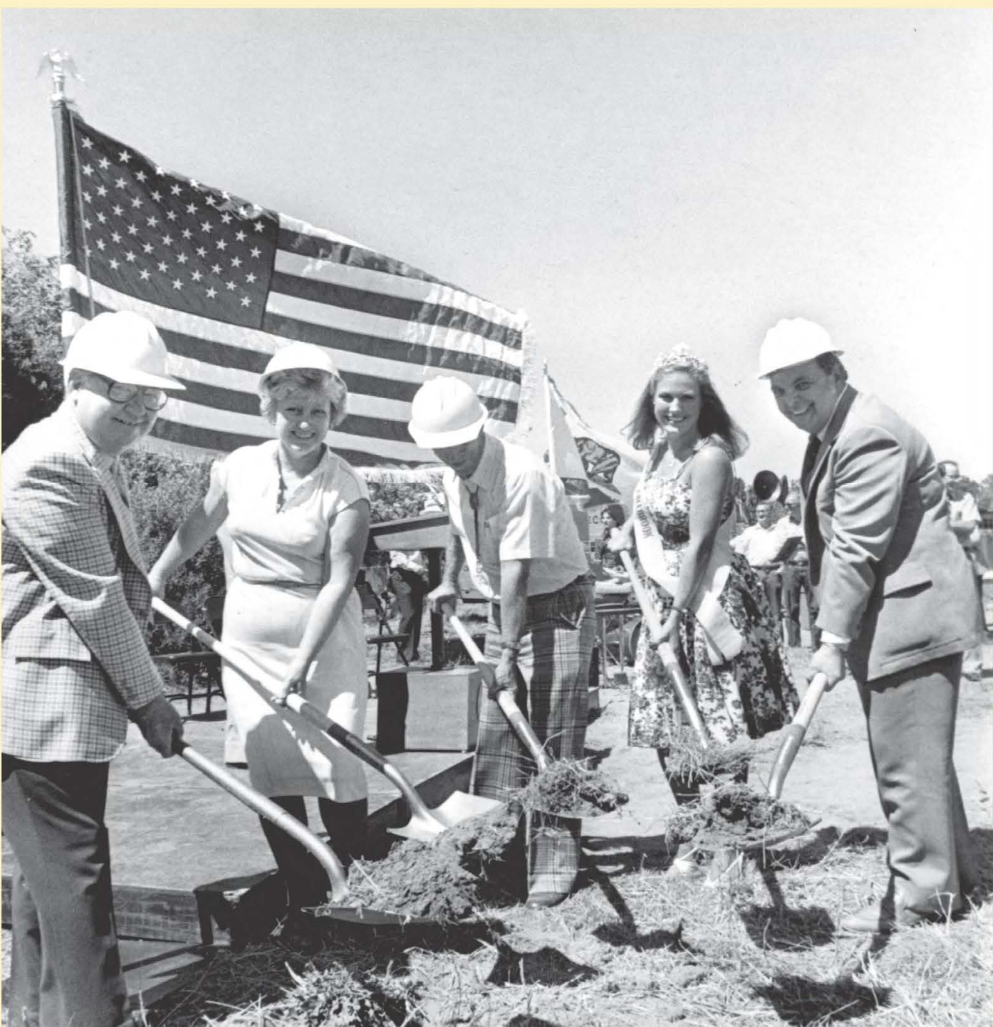
Ground breaking at Fallbrook Community Center was held in 1980, with DPR Director Lloyd Lowrey participating.
