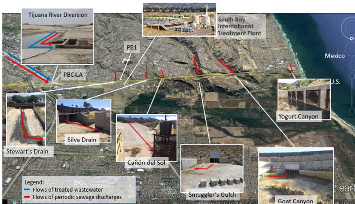
Figure 1. Dry-weather Flow Infrastructure in the Tijuana River
