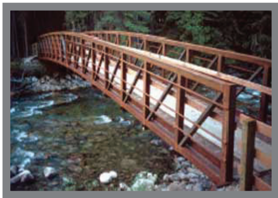
Bridge with 5% camber and "rub rails" 2
