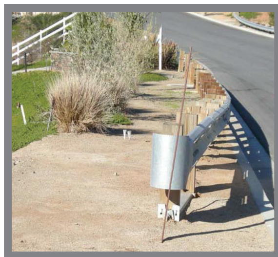
Guard Rail End encroaching into Pathway
