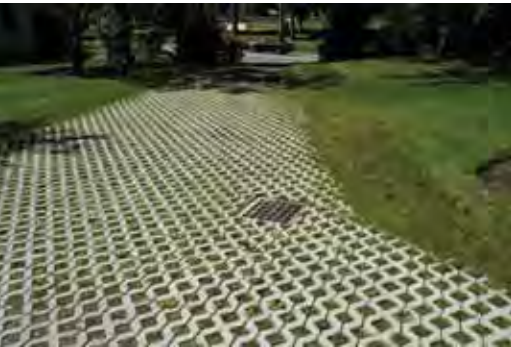
Pervious pavement captures storm-water and allows it to seep into the ground which then recharges groundwater, reduces stormwater runoff and meets the EPA stormwater regulations.
