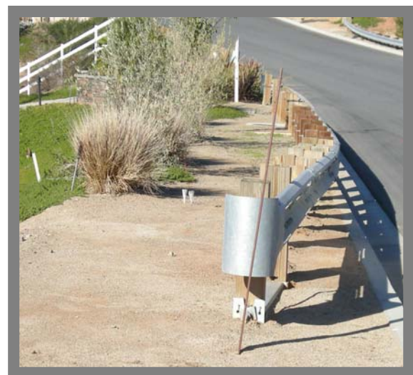
Guard Rail End encroaching into Pathway
