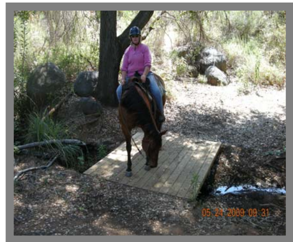
New installed Puncheon being tested in Lakeside
