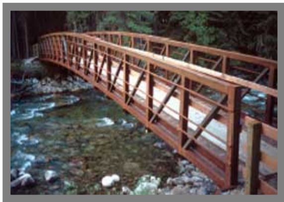
Bridge with 5% camber and "rub rails" 2
