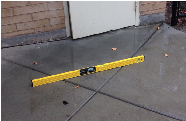
NON COMPLIANT - SLOPES EXCEEDING THE ALLOWABLE % PER CODE
