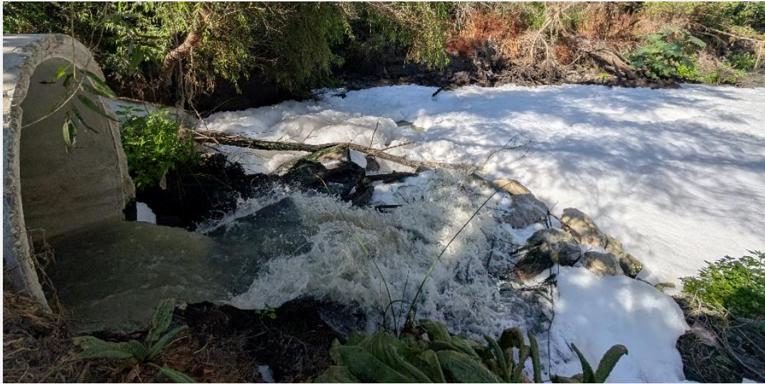
Culvert discharge point and foaming downstream in scour pool. Photo date: 8/27/2025.
