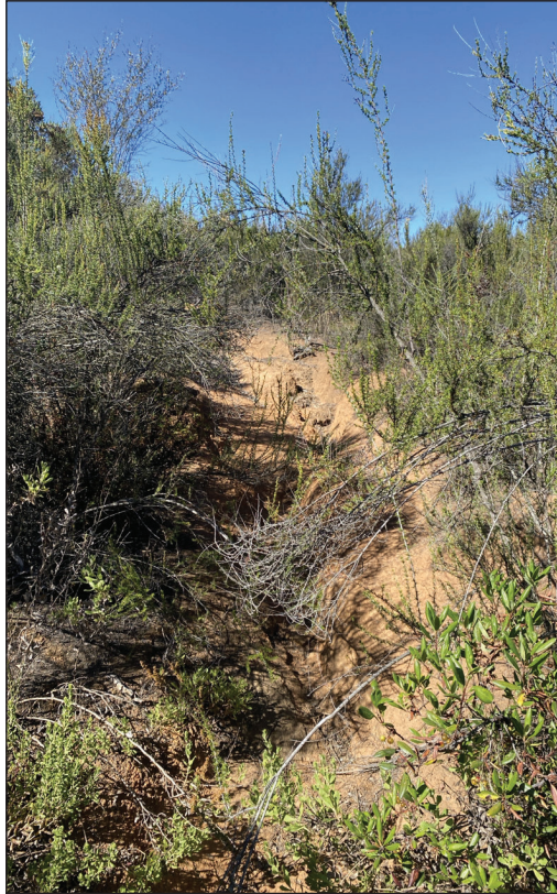
PHOTO 4: Significant erosion adjacent to the trail in the southern portion of the preserve.
