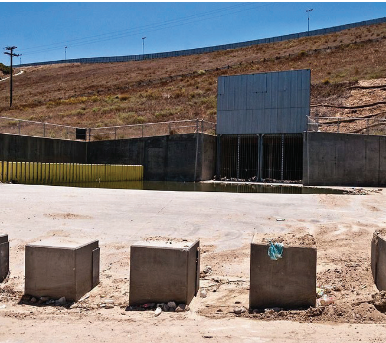
Figure 6: Smuggler's Gulch Diversion Structure
