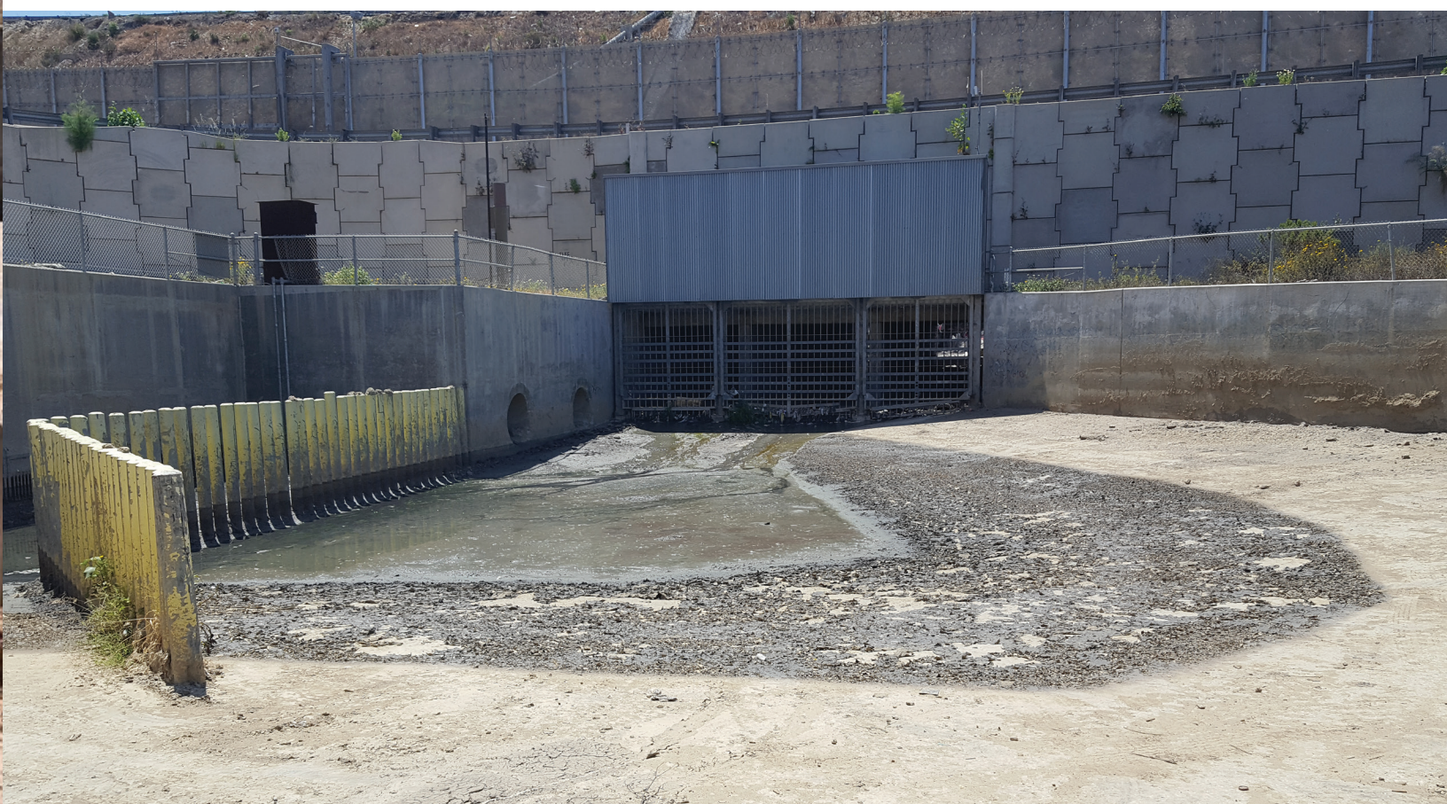
Figure 7: Goat Canyon Diversion Structure
