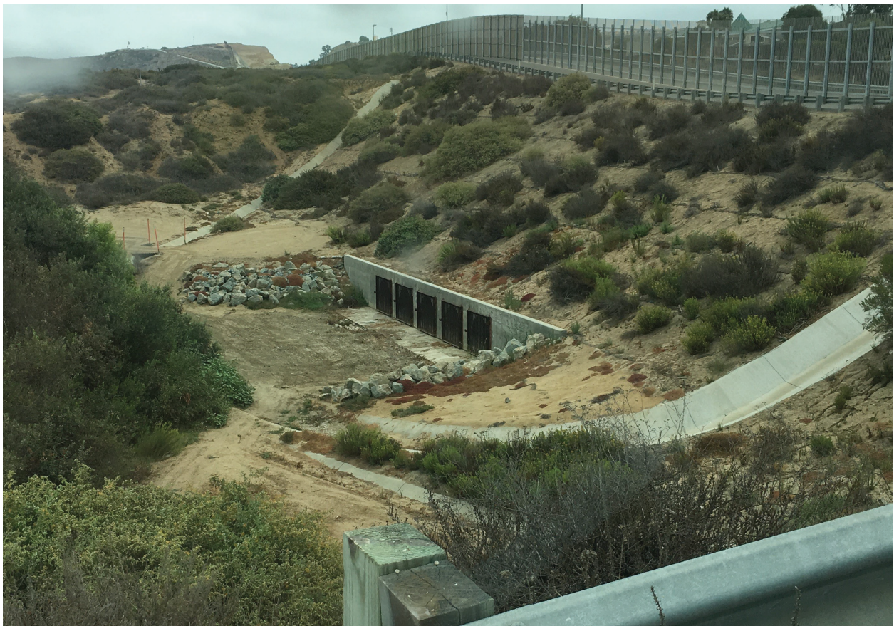
Figure 9: Yogurt Canyon Culvert
