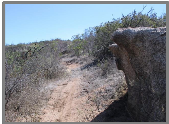
Figure 1. This narrow multi-use trail follows the contour, has an appropriate cross-slope, has a sustainable grade, uses a large rock as a control point, and boasts good line of sight for trail users.
