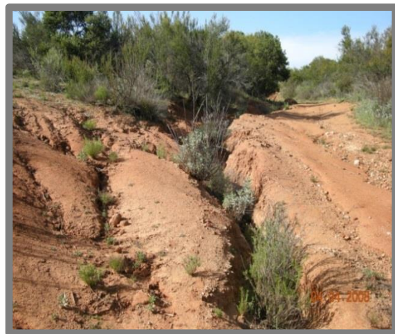
Figure 19. Typical Erosion of a fall-line trail alignment.
