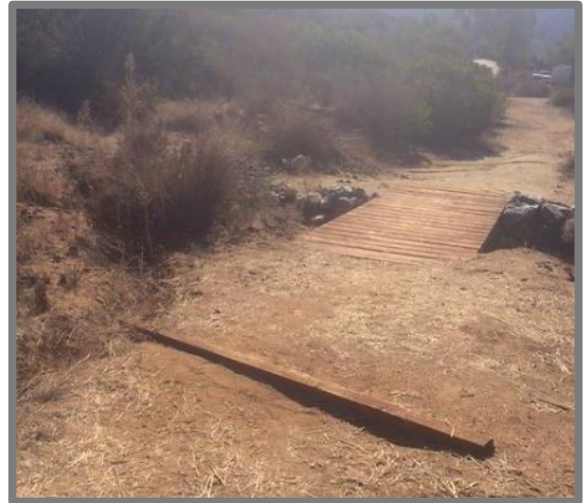
Figure 23. Avoidance of water bar results in “trail creep.”
