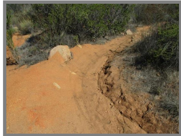
Figure 21. In-sloped turn on a multi-use trail showing erosion and breakdown of the berm; silt build-up on the downhill side does not allow the water to drain off.
