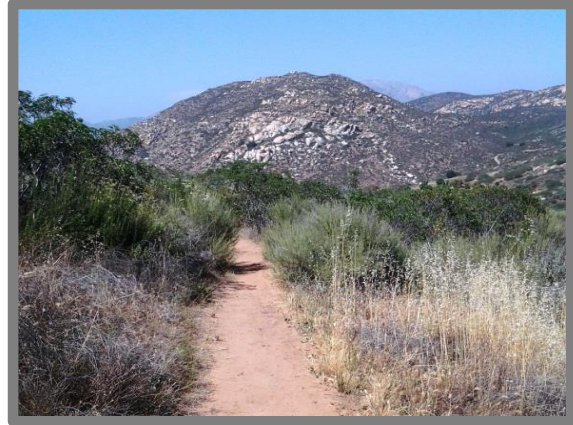
Figure 4. Picture of a sustainable multi-use trail including some characteristics listed above such as: less than 10% grade, good sightline, narrow tread.
