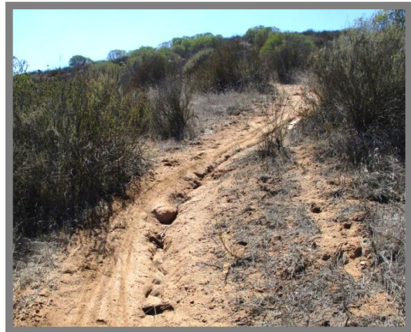
Figure 5. Example of a trail that was not designed with sustainability in mind: no out-slope, an unsustainable grade, shows evidence of trail creep/trail widening, trenching of centerline, lack of water diversions.
