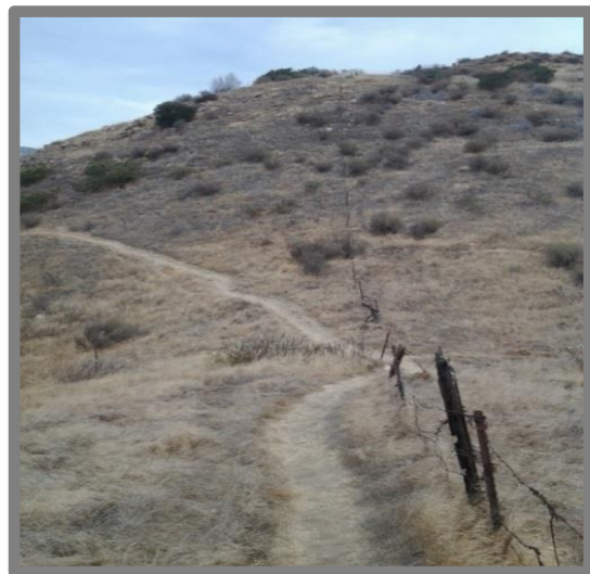
Figure 14. This user created trail has minimal grade deferential, follows the land contour, has a good sight line and cross slope, and has a narrow tread.
