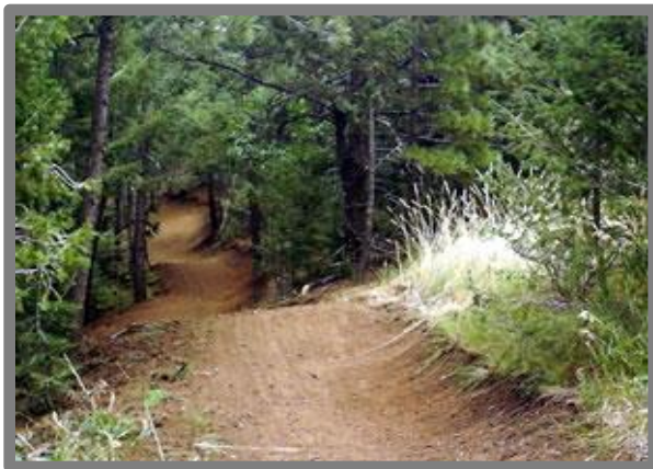
Figure 8. Curvilinear trail with good cross slope and rolling grade dips. Using the trees as control points creates a sustainable trail with minimal maintenance requirements. Photo used with permission from Arrowhead Trails, Inc.
